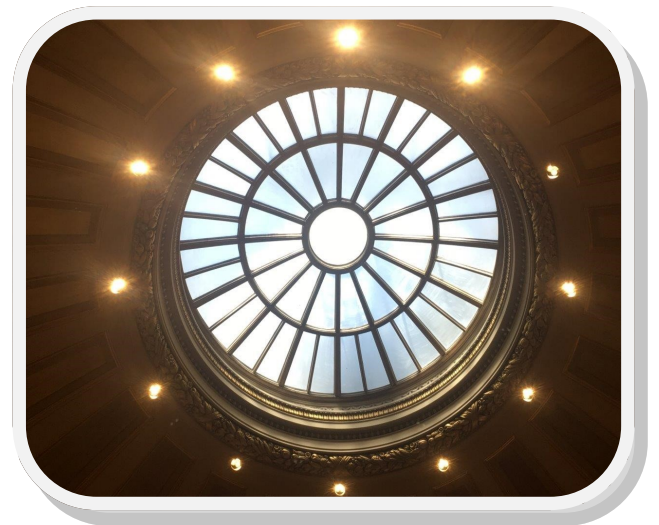
Natural light permeates the refurbished courtroom, giving a sense of what it was like before all buildings were wired for electricity. (Steve Aggergaard photo.)
